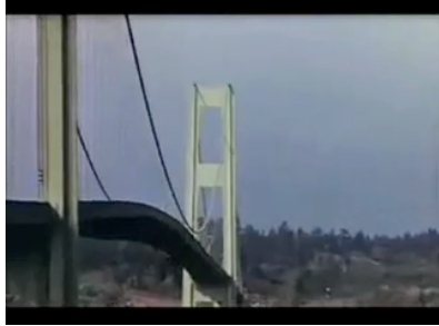
Tacoma Narrows Bridge Collapse
